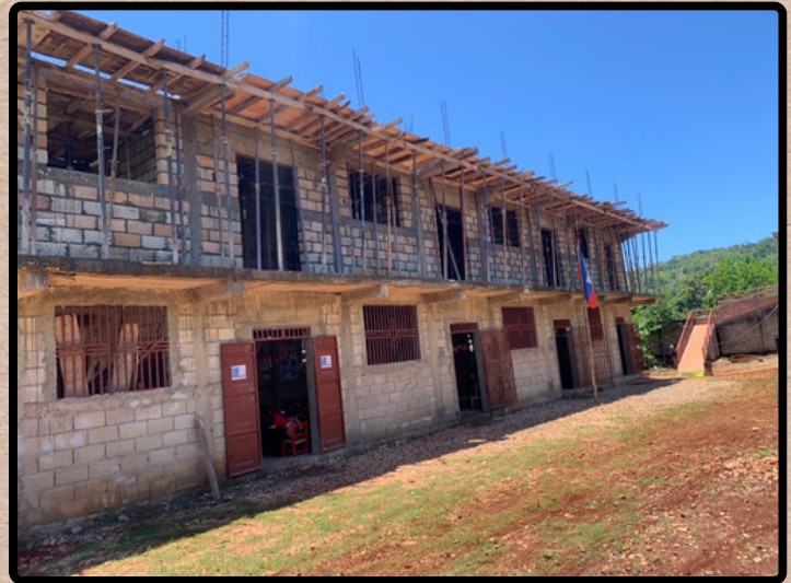
Outside view of the construction's preparation for the slab
