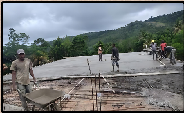
Workers setting up the slab for the 2nd floor of New Hope academy
